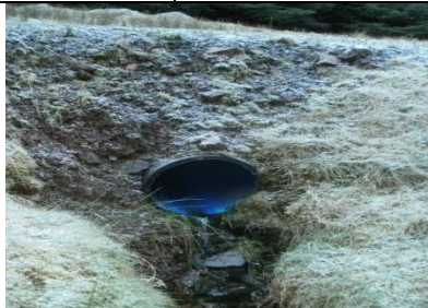
Existing 450Ø HDPE pipe outlet
