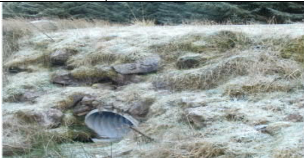
Existing 450Ø HDPE pipe inlet
